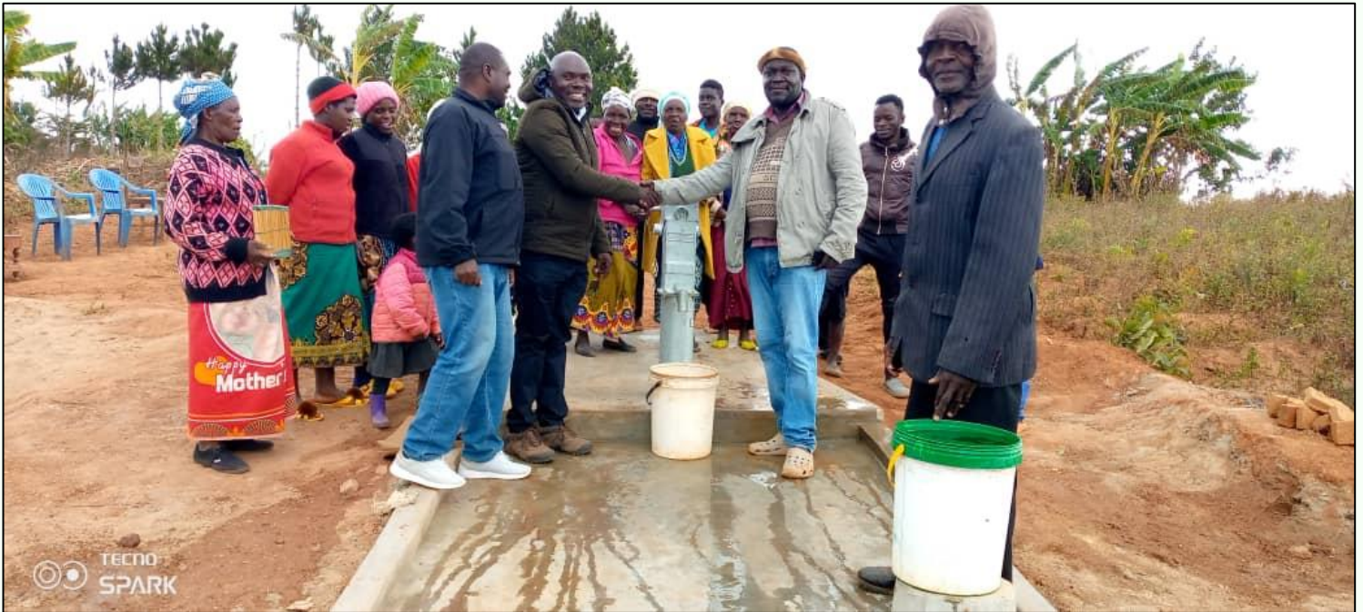
The official handshake between Pastor Dennis Singini and the Village Chief during the commissioning of OB 2 Village Well in Mambongo Village, August 28, 2023. Over 900 villagers now benefit from clean water.
